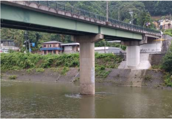
P2橋脚施工前
